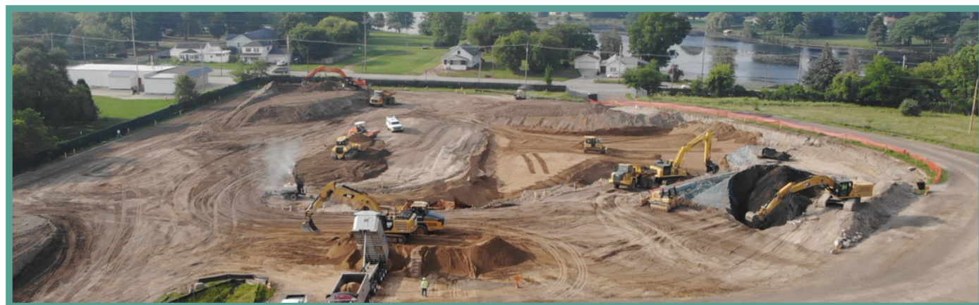
Aerial view of PSA-1 Excavation activities
